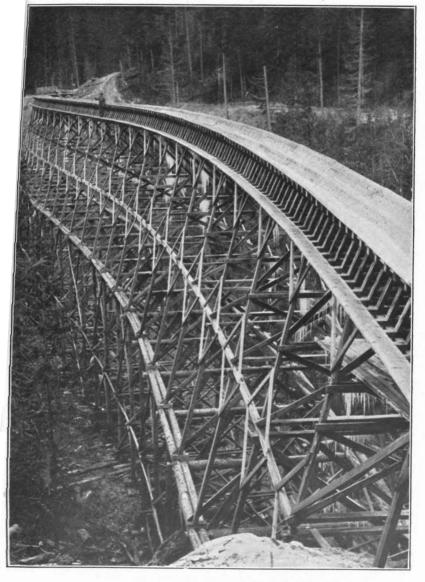
Section of Flume Built and Operated by the Adams River Lumber Co,
